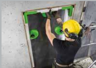
5. Demolding
